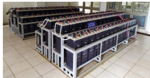
Fig 5 BESS setup in the BTP.
