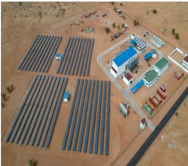
Fig 1. Aerial views of the Kiffa Hybrid Power Plant, © VERGNET © ABC CONTRACTING
