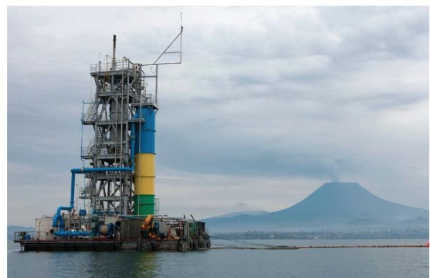
Fig. 4 Pilot exploitation methane to electricity station at Kivu Lake
