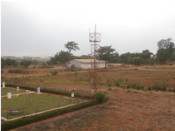
Fig. 2 Mast of the wind data collection of the Ngaoundere Airport
